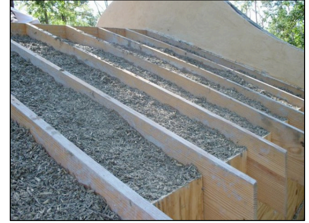
Hempcrete – roof insulation
