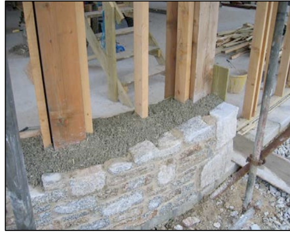
Hempcrete – cast around frame
